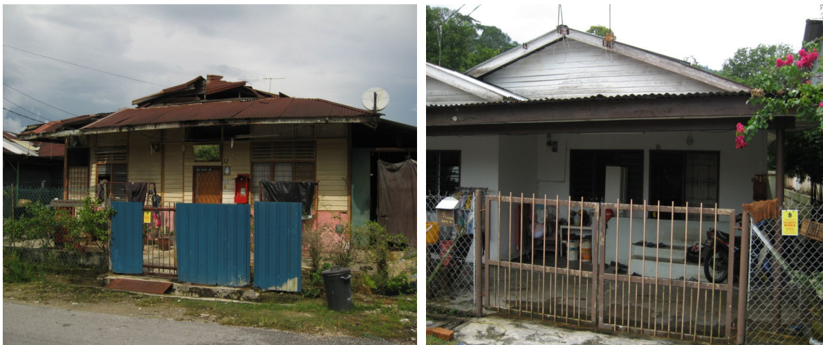
Photo 2: Old and dilapidated house
